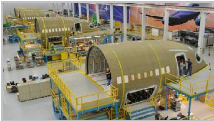
787 Forward Fuselage Systems Installation
