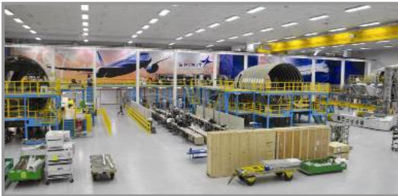
787 Forward Fuselage Systems Installation Facility
