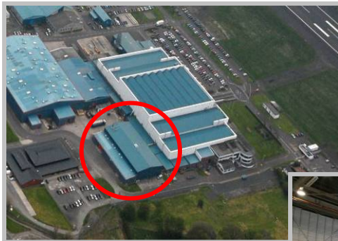
European MRO Facility – Prestwick International Airport
