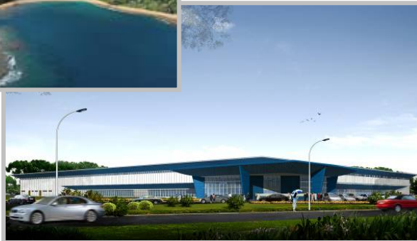
Spirit Malaysia Facility
